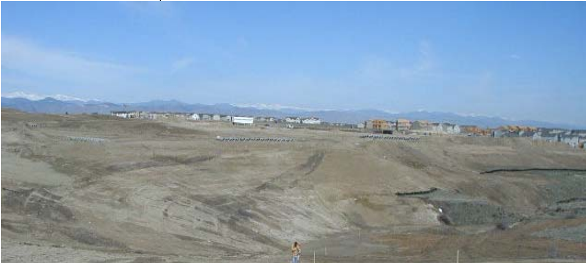
Large areas of disturbance create huge potential for erosion and sedimentation; limiting the area of disturbance substantially reduces the problem.
