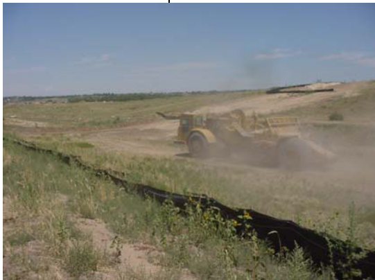
Control of airborne emissions is to be addressed in the GESC Plan and may be subject to additional State regulations.
