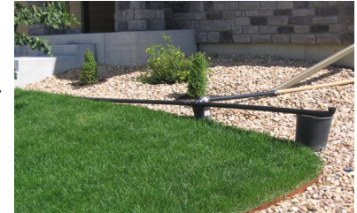
Modifications done to use sump water across green area
