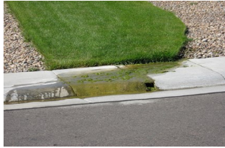
Excessive water flowing over sidewalk
